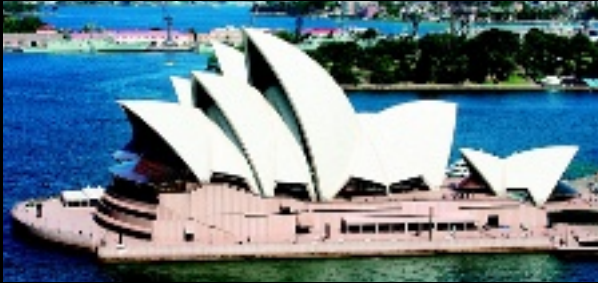
The powerful geometric forms of Sydney Opera House. © Michael Moy Idea to Icon
