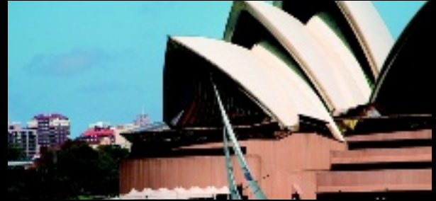
The podium is clad in earth-toned panels © Michael Moy Idea to Icon
